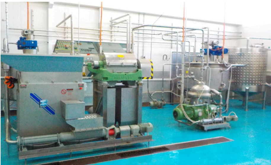
The state of the art compact organic oil processing facility at Mantzaris fisheries in North Geelong
